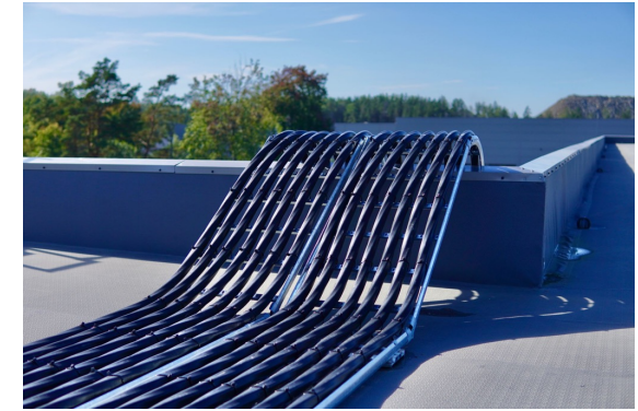
1 km AC kabler
